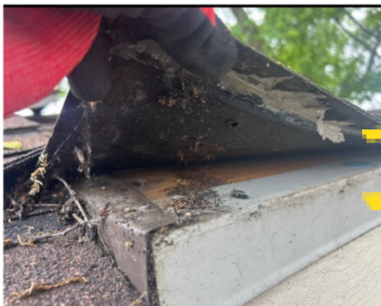
No felt paper on the front portion of the house
